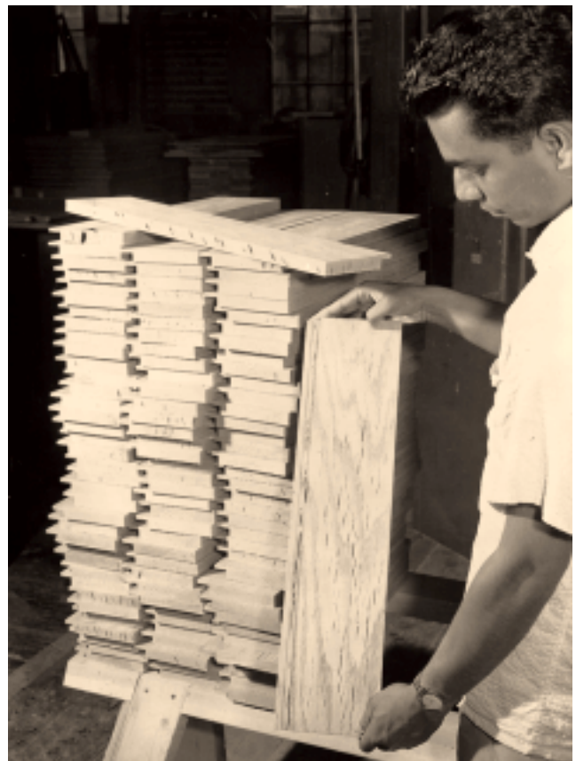
Figure 9.1—Extensive surface checking in oak lumber.
